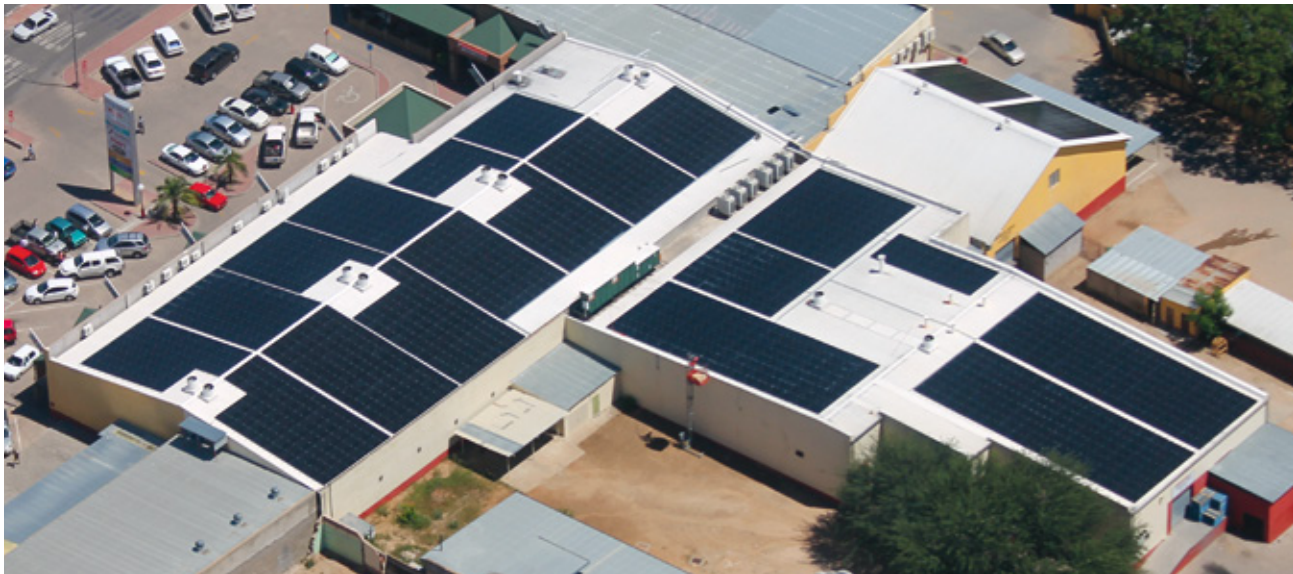
Namibia's first SPAR supermarket to source renewable energy using a rooftop solar energy system. (Image: HopSol)
